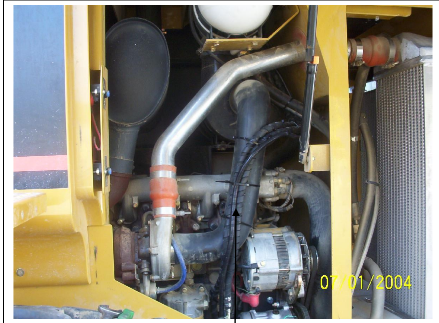
Hoses running up to the condenser.
