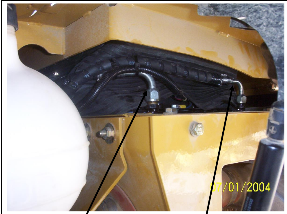
13/32" fitting at condenser
