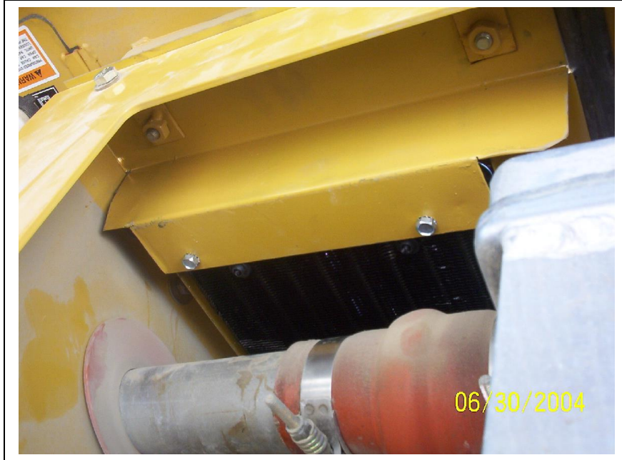
Right side of the condenser mounted in place
